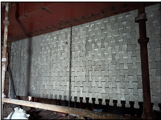
Fig. 1: Baffle wall precast
