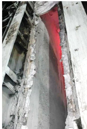
Fig. 1. Fused Silica Gunning Repaired Heating Wall
