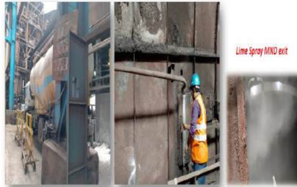
Coating trial at Sinter plant -2 TSI
