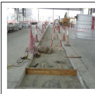
Fig.1 Casting of High Strength Floor
