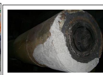
Fig.3 Repaired burner tip with Topcrete
