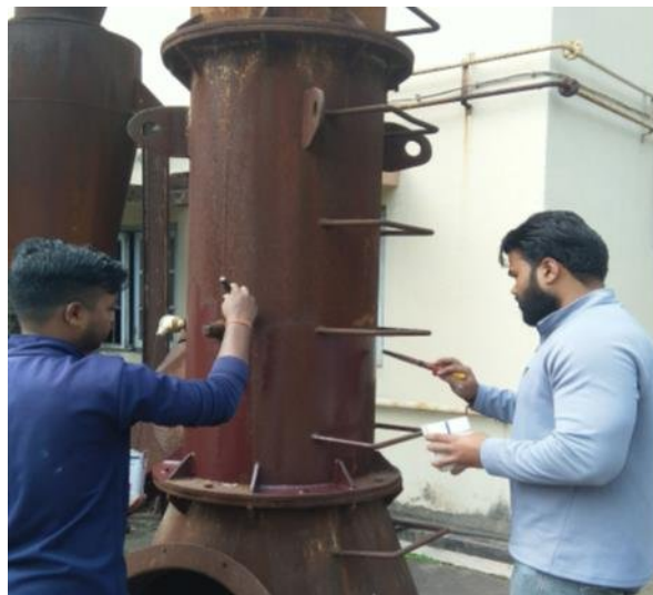
Fig. 1: Ceramic Primer application on rusted steel
