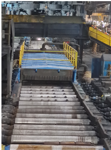
Fig. 1: Primary descaler hood
