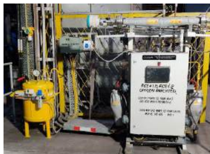
Fig. 1: Laser based oxygen analyser
